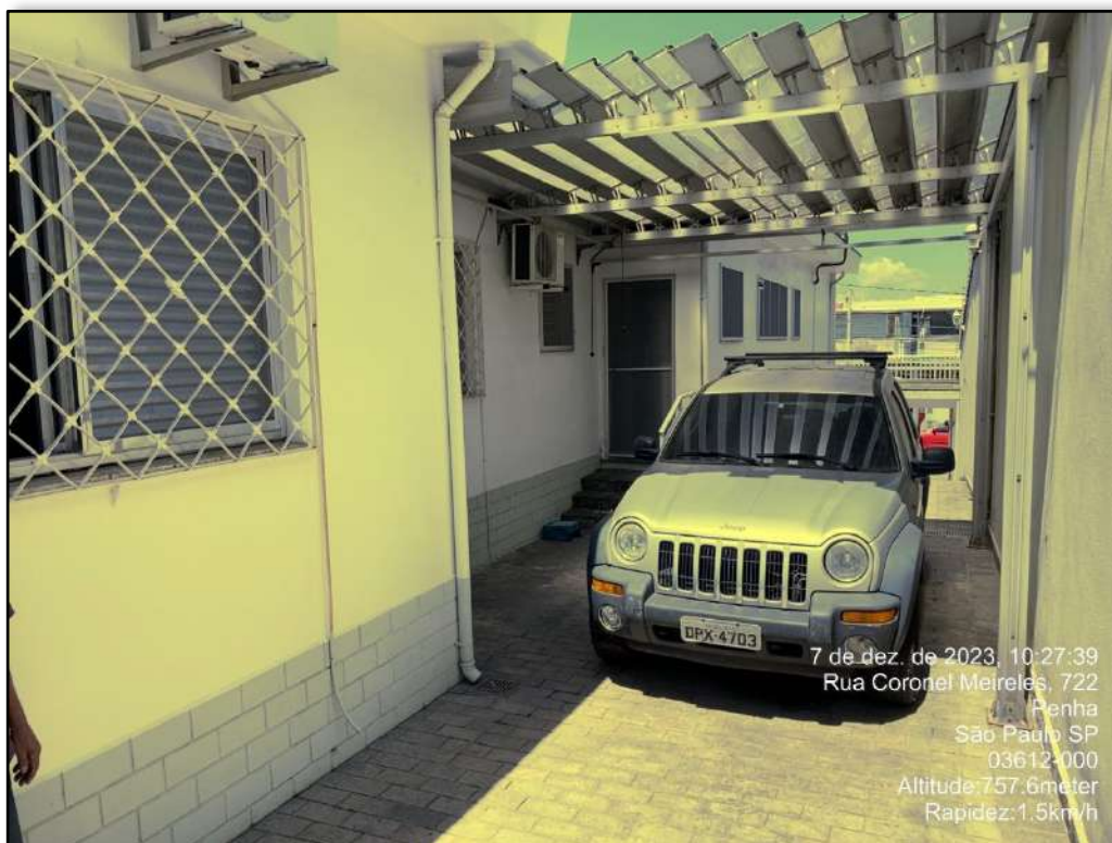
40 – QUINTAL LATERAL VISTA INTERNA 2
